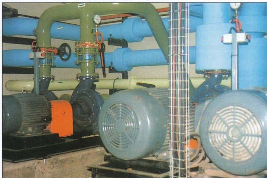
Chilled water and condenser water pumps in the plant room.
